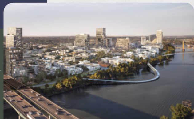
An artist's rendering shows planned development and waterfront features in the City of West Sacramento; FAR RIGHT Oceanside is part of the Innovate78 partnership.
